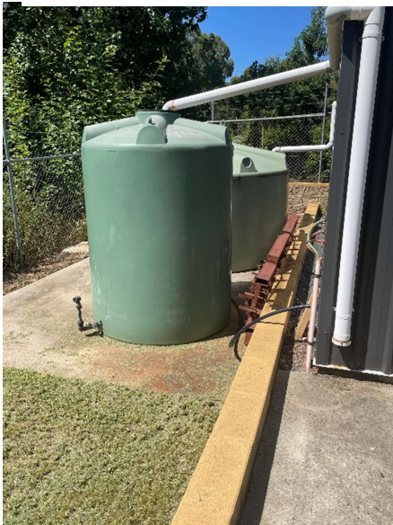
The water supply is via rainwater tanks. Water to the steaming bays is via a pump from the tanks to a tap at the services point.
