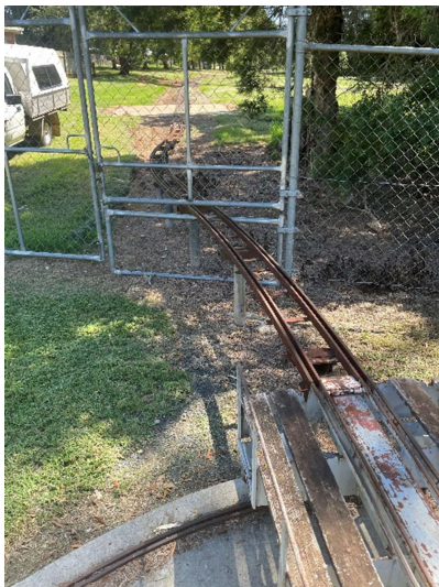
Access from the compound out onto the main branch line. Visitors, please note at this section the 5" gauge is centred in the 7 ¼" gauge and changes on the main line. To achieve this, you travel through a 5" to 7 ¼" transfer point , drivers need to check the positioning of the point before traversing through.
